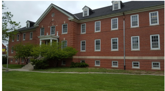
Figure 1 Building # 5 Future occupancy by Aging Partners
